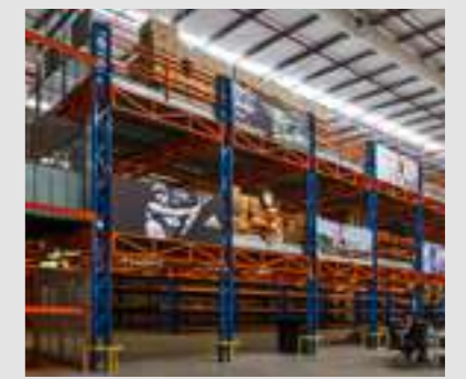
RACKS C/ PASARELA
